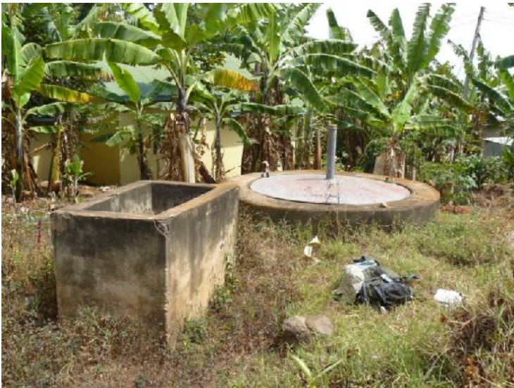
Biogasanlage Nyakahanga Hospital
