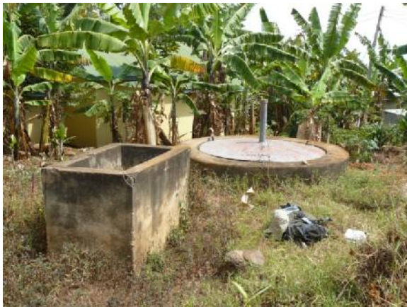
Biogasanlage Nyakahanga Hospital
